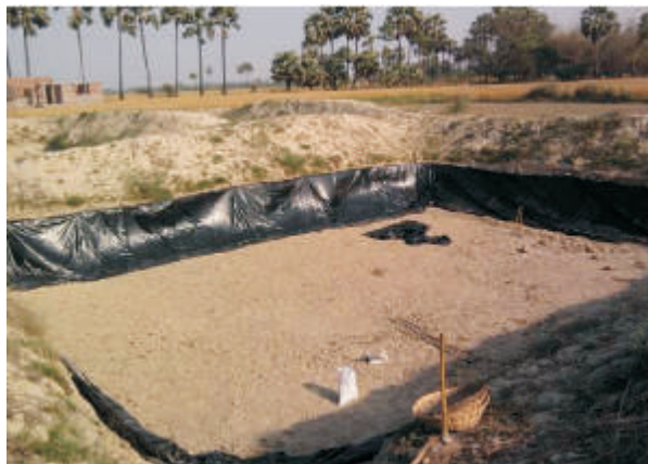
HDPE lined pond preparation
