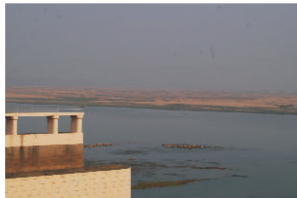
River bed below Indrapuri barrage
